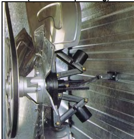
Centrifugal shutter system (fan is not operating)
